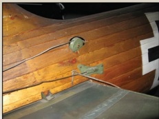
Tailplane attachment brackets and elevator control cable pulley.
